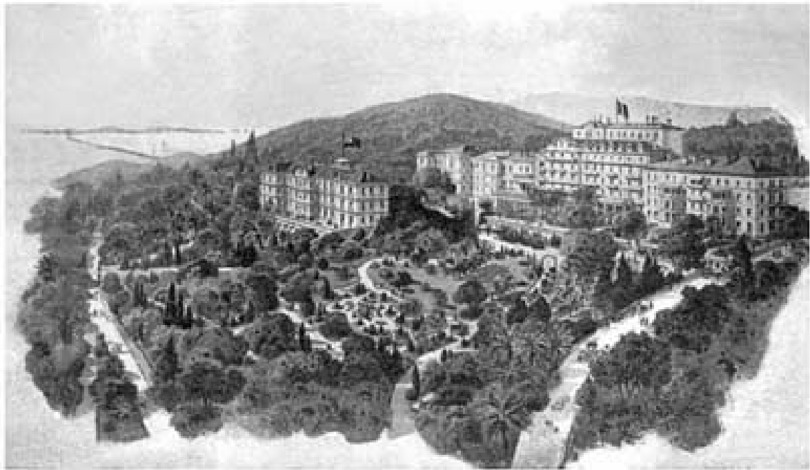
GENERAL VIEW OF HOTELS
